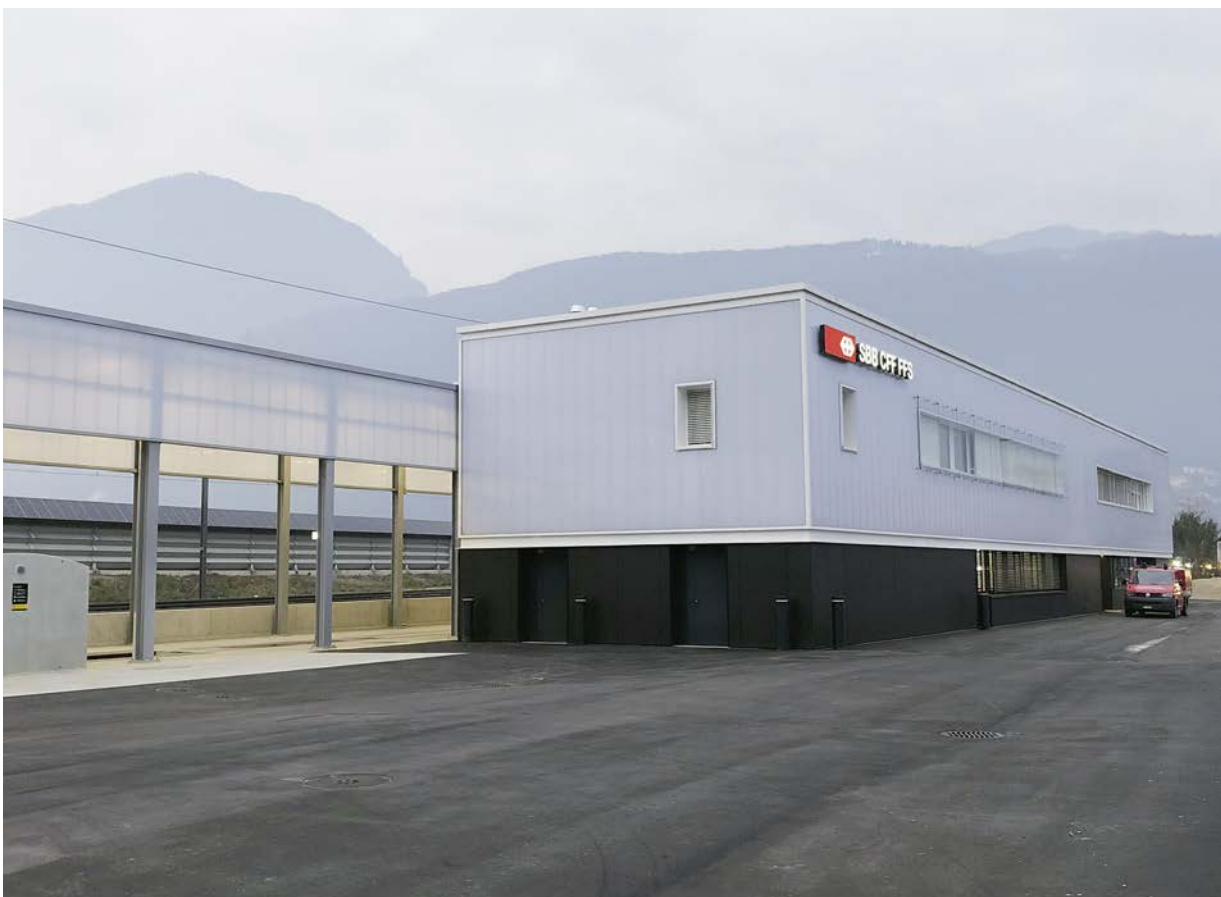
NEAT, Interventionszentrum Melide.
